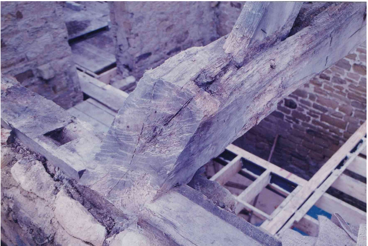
Figure 21: Stable block: tie beam of principal rafter (1995)
