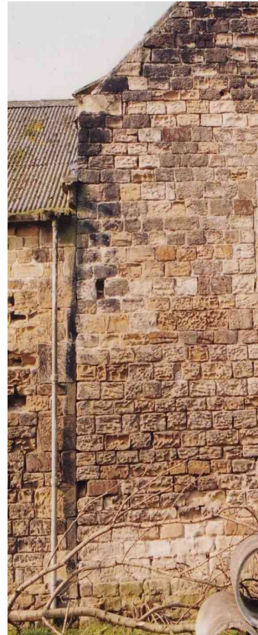
Figure 18: Barn - Stable joint and quoins E elevation (1995)
