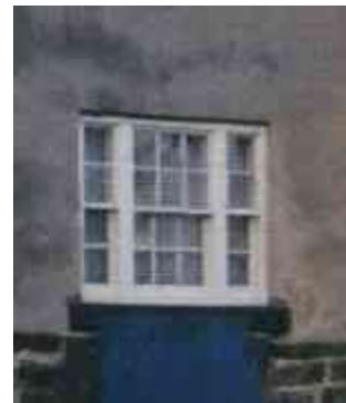
Figure 8: 'Cottage' rear window (1995)
