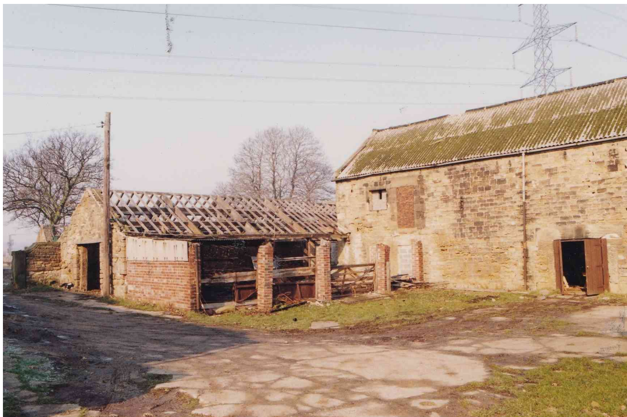
Figure 19: W end of barn and cart shed (1995)
