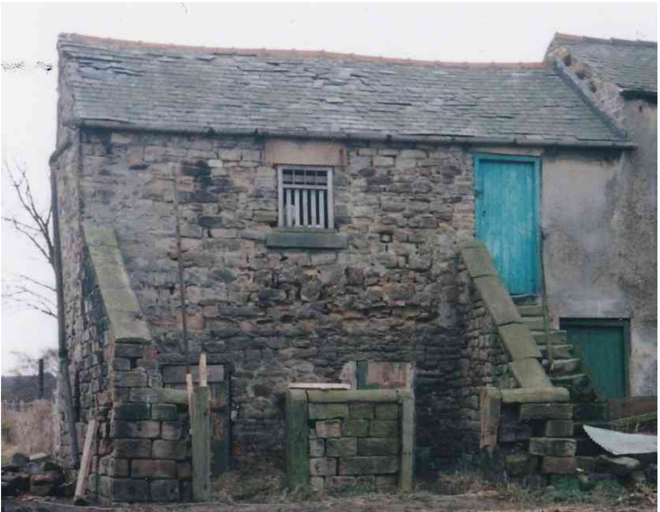
Figure 14: Store / Piggery N elevation (1995)
