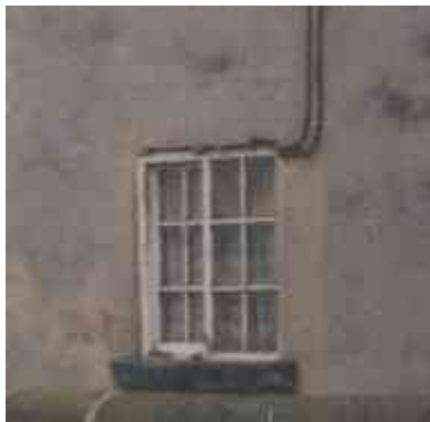
Figure 7: House rear window (1995)
