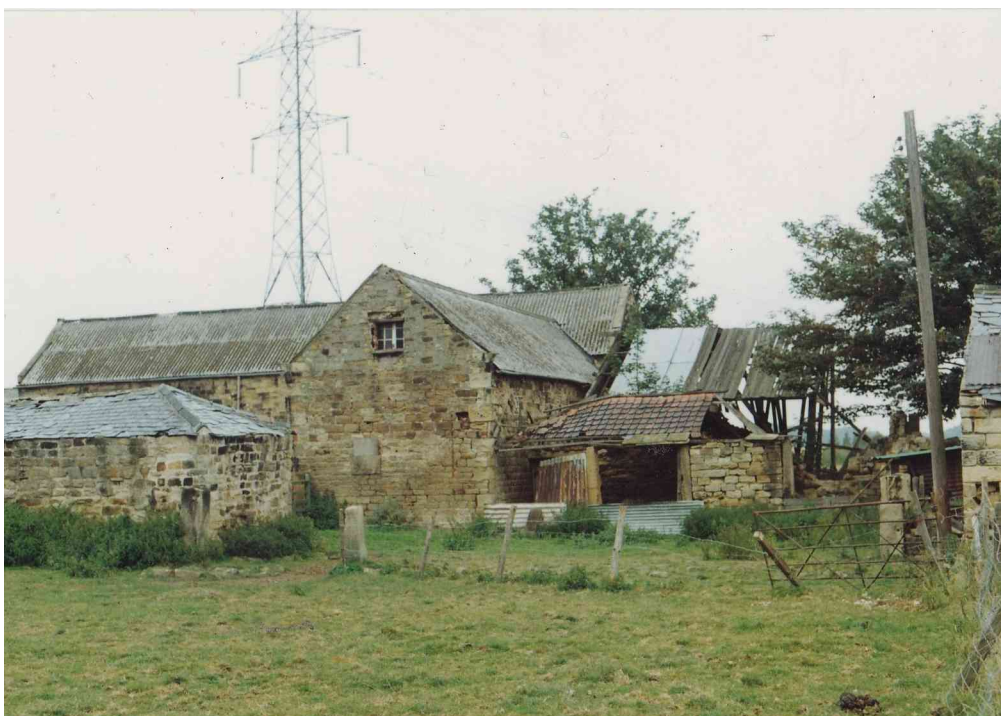
Figure 20: Stable block viewed from SW (1995)
