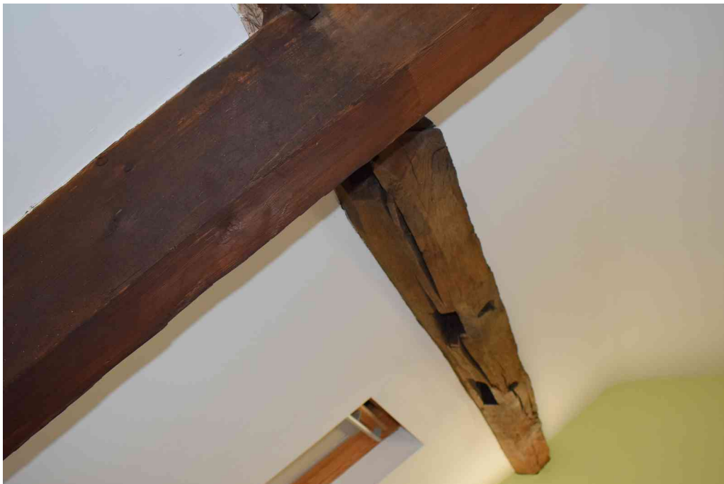
Figure 5: Photo of timber reused as a purlin showing empty mortices and pegholes.(October 2022)
