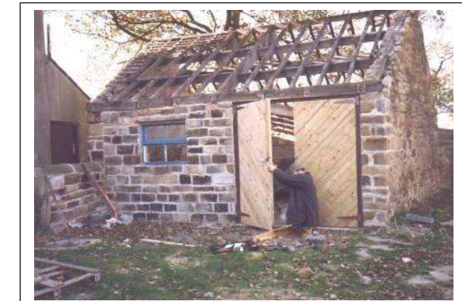
Repairing a garage to create a store for the stonemasons.
