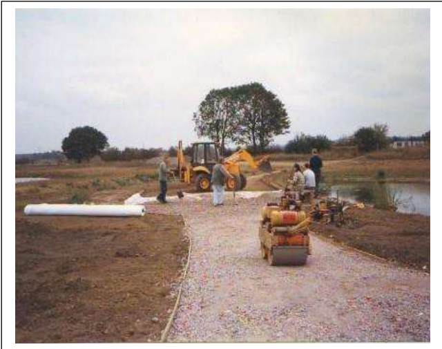
Footpath construction in themed area October
