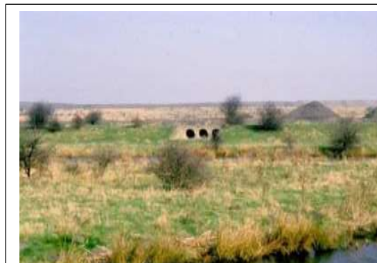
Flood Defence outlet Flap Valves to River Dearne
