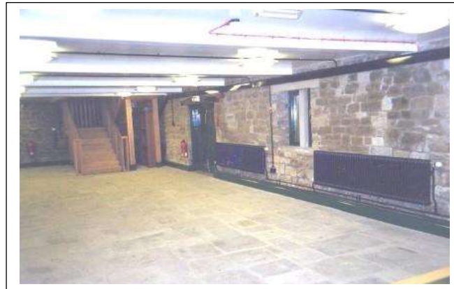
Visitor Centre Ground Floor January
