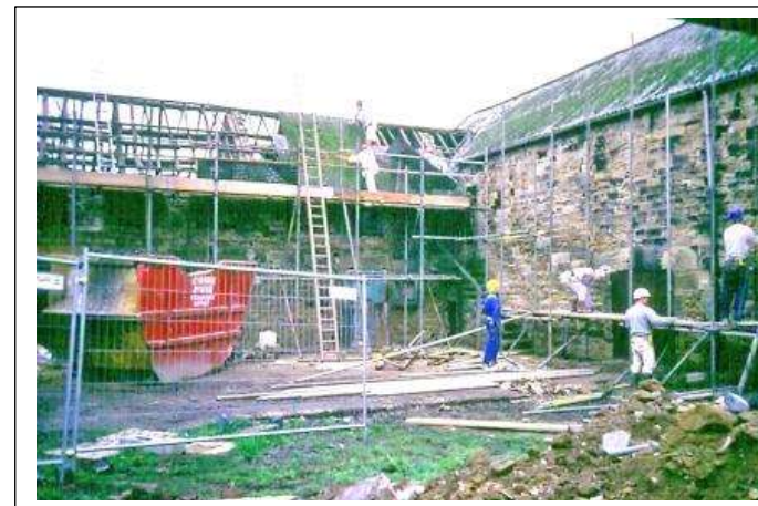
Scaffolded barn with roof works under way December
