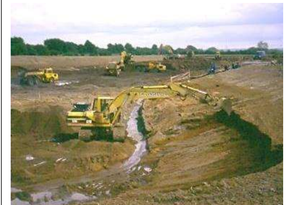
Reservoir excavation May
