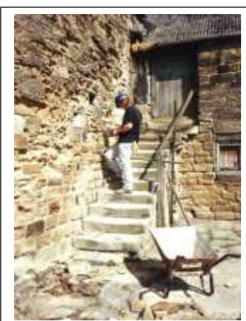
Barn wall re-pointing August
