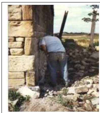
Stonework repairs August
