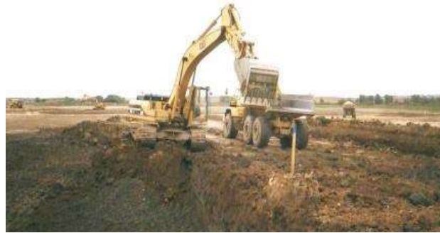
Excavation in the main lake in September
