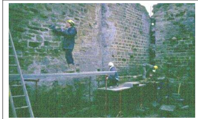
Repointing external walls of barn
