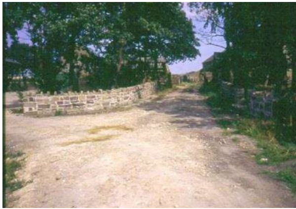
Repaired and rebuilt stone walls in the farmyard
