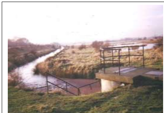
Main Drain & Flood Defence outlet pump
