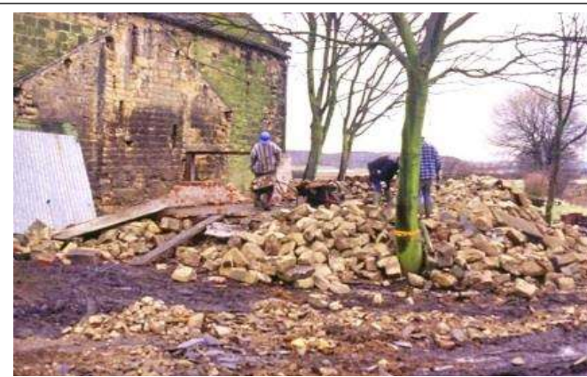
Stonework repairs around the barn.
