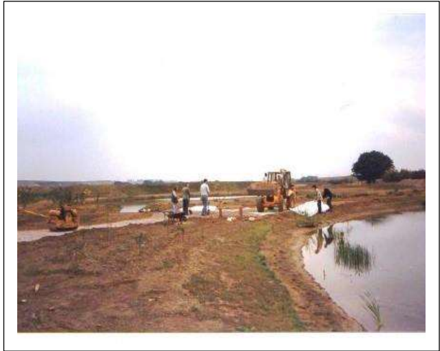
Footpath construction in themed area October
